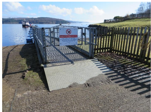
6. Access to alternative jetty supervised access only.
