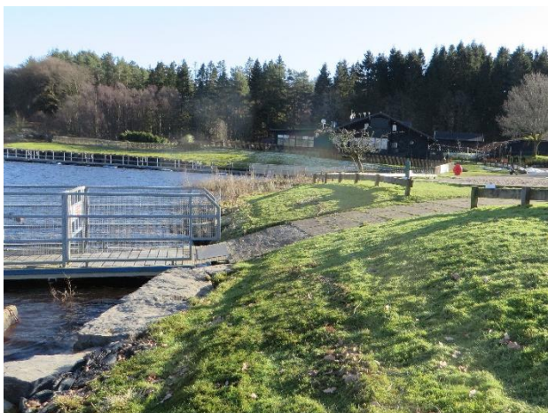
5. Steep access to jetty with hoist supervised access only.
