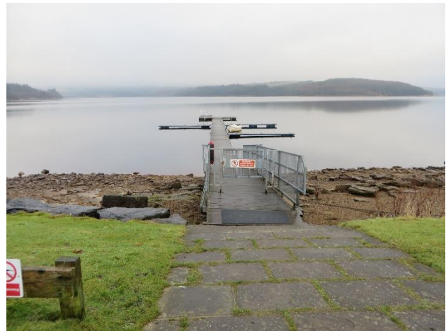
4. Access to jetty supervised access only.
