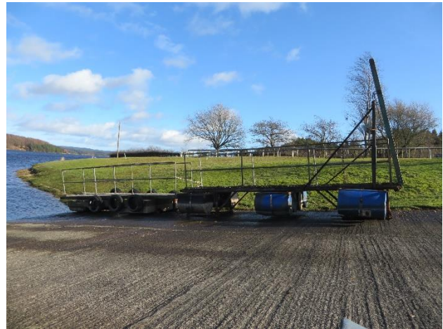
2. Slipway tamped concrete surface.
