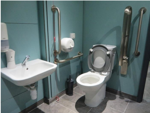
1. Accessible WC/shower room.
